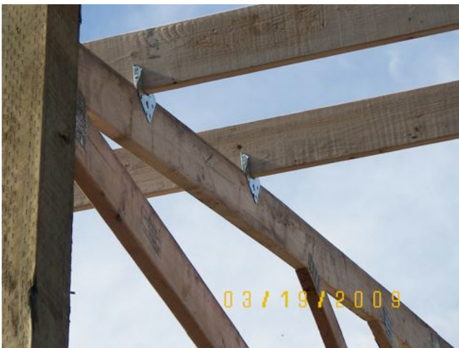
H-1 installed on inside of end truss
