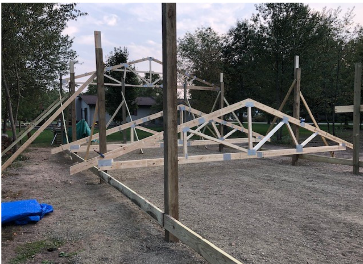
Raised Heel Trusses
