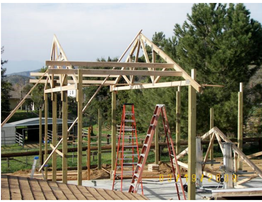
Figure 55-7 Eave Strut Overhang
