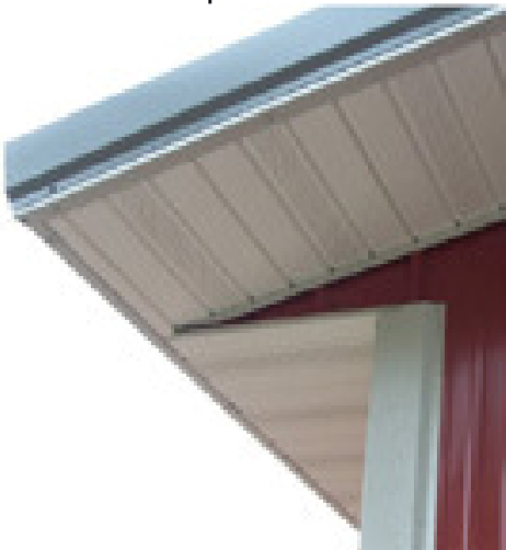
Figure 55-42 Fold Over Top Of Corner Trims
